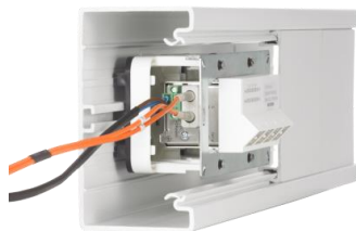
Installed on a C-profile anchor rail in a tehalit duct
