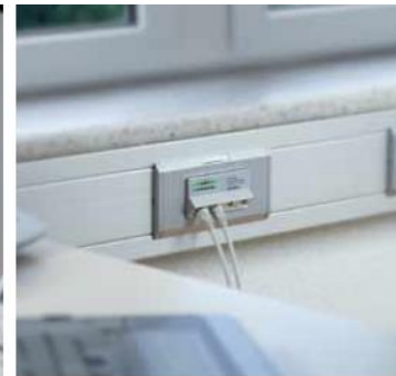
Cable trunk installation
